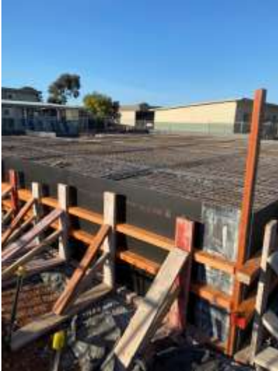
Getting ready for the concrete pour for the first half of the Junior Learning Building.
