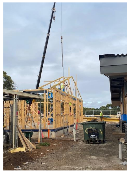
Roof trusses were being installed today.
