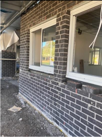
Brickwork is almost finished on the ground floor of the SLB.
